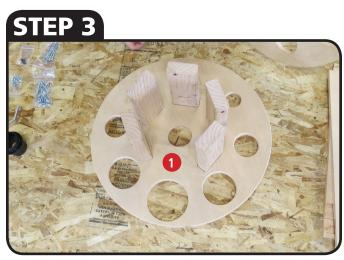
AFTER 2x4s ARE CUT TO SIZE PLACE INTO POCKETS ON INNER WHEEL
